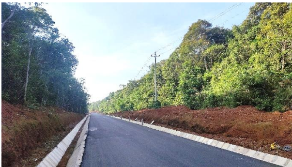
Newly paved road
