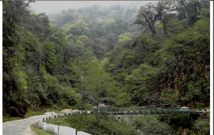
Bridge on the Lingmethang Road
